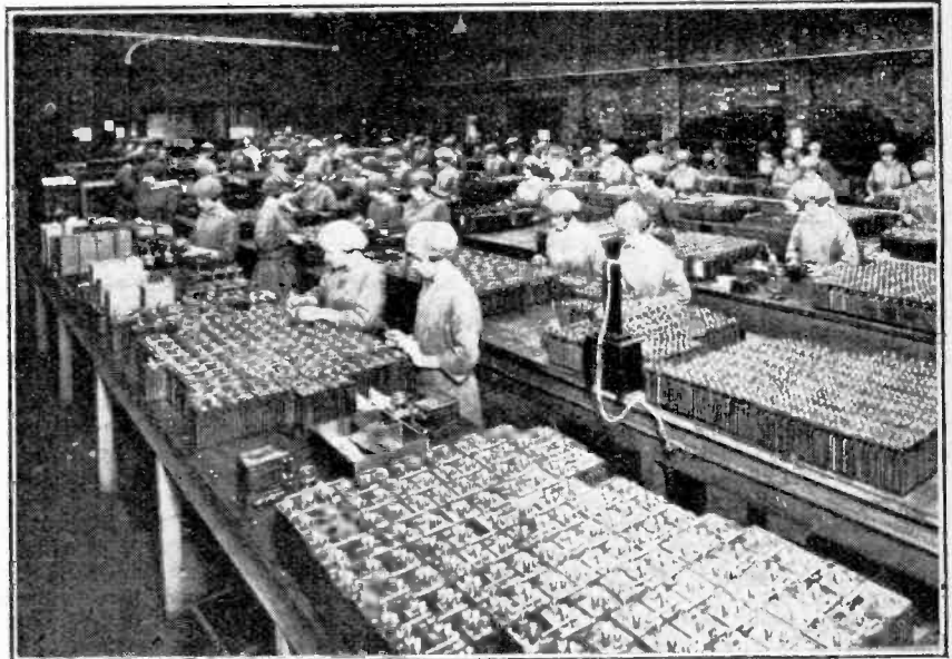
A section of the Exide works showing the assembling of cells.
